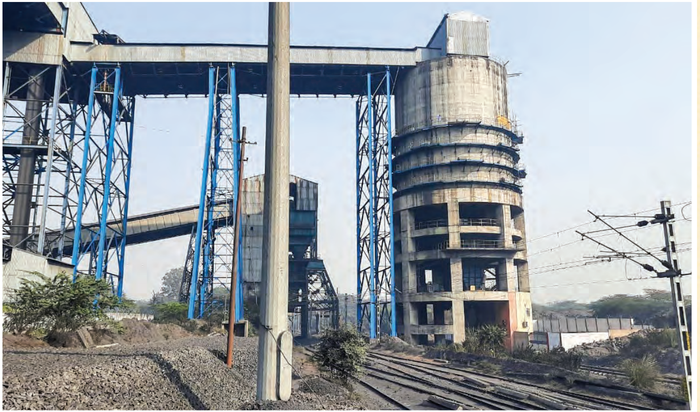
Commissioning of Krishna Shila Project by HEC in NCL
