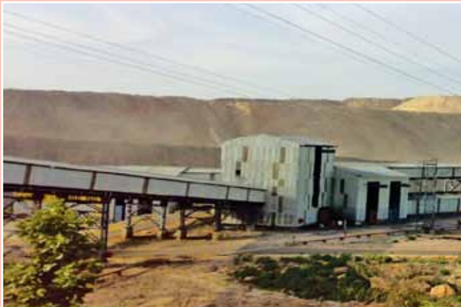
Coal Handling Plant at Nigahi, Singrauli, Northern Coalfields Limited.
