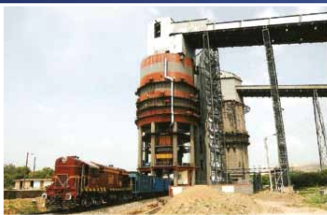
Silo, Ore Bedding and Blending Plant, RSP Rourkela
